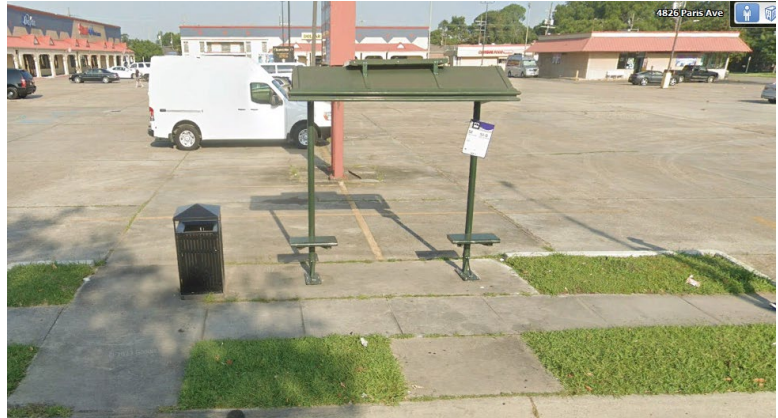
Photo shows transit stop at Mirabeau Ave and Paris Avenue (southbound).
