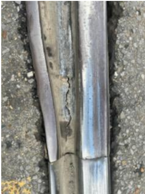
Welding repairs in Harmony Circle
